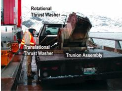
The trunnion assemblies are loaded on a truck for transport to the repair shop.
