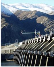
A gantry crane erected on the spillway at Priest Rapids Dam in Washington State (USA) is used to install rebuilt trunnion assemblies at each of the dam's gates.
