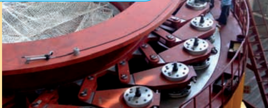
Installation of Alstom hydro generator in Three Gorges dam
